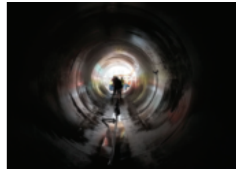
Finished sewer tunnel. Looking towards Kaneohe tunnel shaft.
